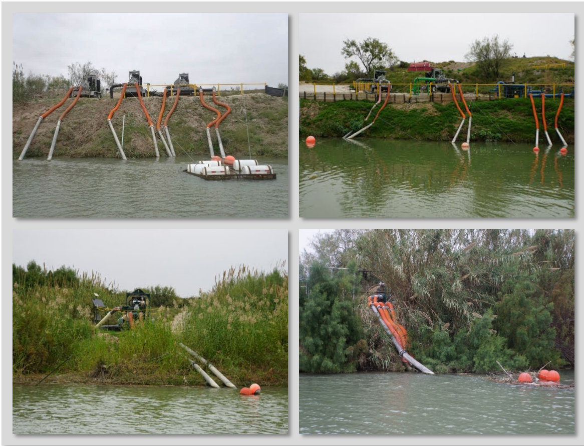
Figure 9. Diesel pumps 95 operating on the Rio Grande to extract water for mining purposes in Webb County; photos courtesy of Colin McDonald 96
