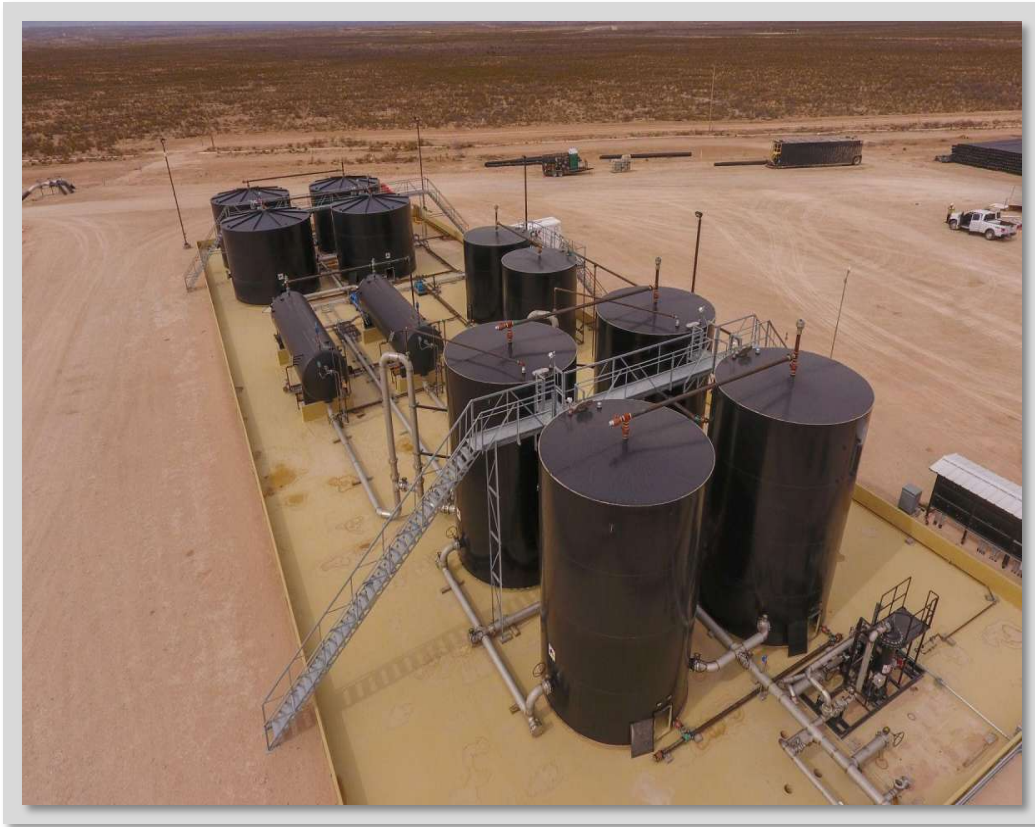
Figure 10. A salt-water disposal (SWD) facility located in the Permian Basin, West Texas; photo courtesy of the Houston Chronicle
