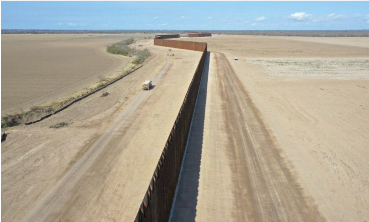
FIGURE 1: REPRESENTATIVE IMAGE DEPICTING THE SCALE OF THE WALL, MAINTENANCE ROAD, AND PATROL AREA COMPONENTS OF THE PROPOSED SYSTEM. SOURCE: HTTPS://WWW.CBP.GOV/DOCUMENT/ENVIRONMENTAL-ASSESSMENTS/BORDER-BARRIER-AND-WATERBORNE-BARRIER-SYSTEM-WEBB-AND-ZAPATA
